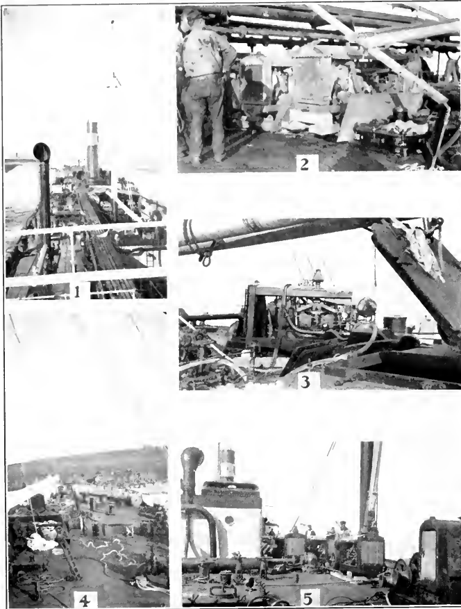
(1) View along the deck of the Tamiahua showing the heavy seas breaking over the stern. (2) and (3) The engine-driven air compressors which were used for filling the cargo tanks and supplying air for the operation of the steam steering gear. (4) View from the bow of the Tamiahua showing the lines to the bluff. (5) A view of the deck with some more of the engine driven compressors in the foreground.
